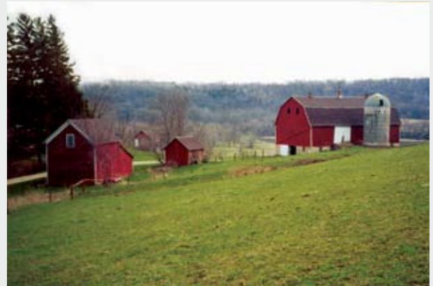
This sample application was developed for the barn on the right pictured above. The image below, left, shows a deteriorated section of the limestone foundation.
